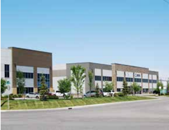
Photos: Examples of Industrial General
