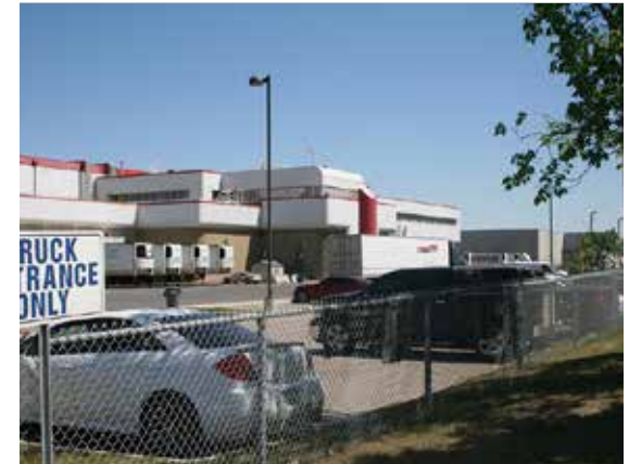
Photos: Examples of Industrial General
