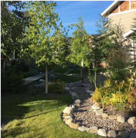
Photo: This neighbourhood housing development incorporates stormwater collection and filtration infrastructure.
